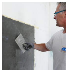
Step 4: Marble effect created through impregnation with MC-Color Proof pure
