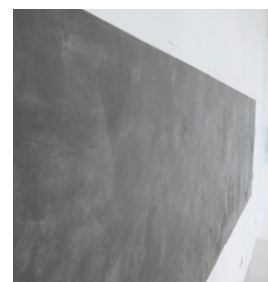
Step 5: Final finish with a second coat of MC-Color Proof pure. And that's it!
