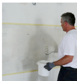
Step 1: Masking and – depending on requirements – priming of the area to be treated.
