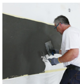
Step 2: Application of the first layer of Emcefix-Spachtel F lang in anthracite grey.
