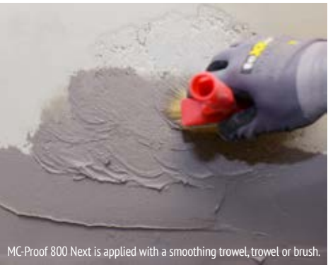
MC-Proof 800 Next is applied with a smoothing trowel, trowel or brush.
