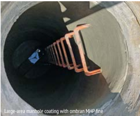
Large-area manhole coating with ombran MHP fine
