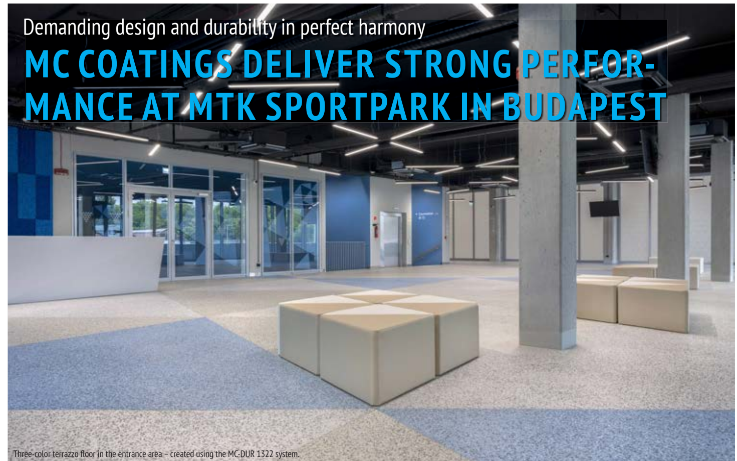
Three-color terrazzo floor in the entrance area – created using the MC-DUR 1322 system.
