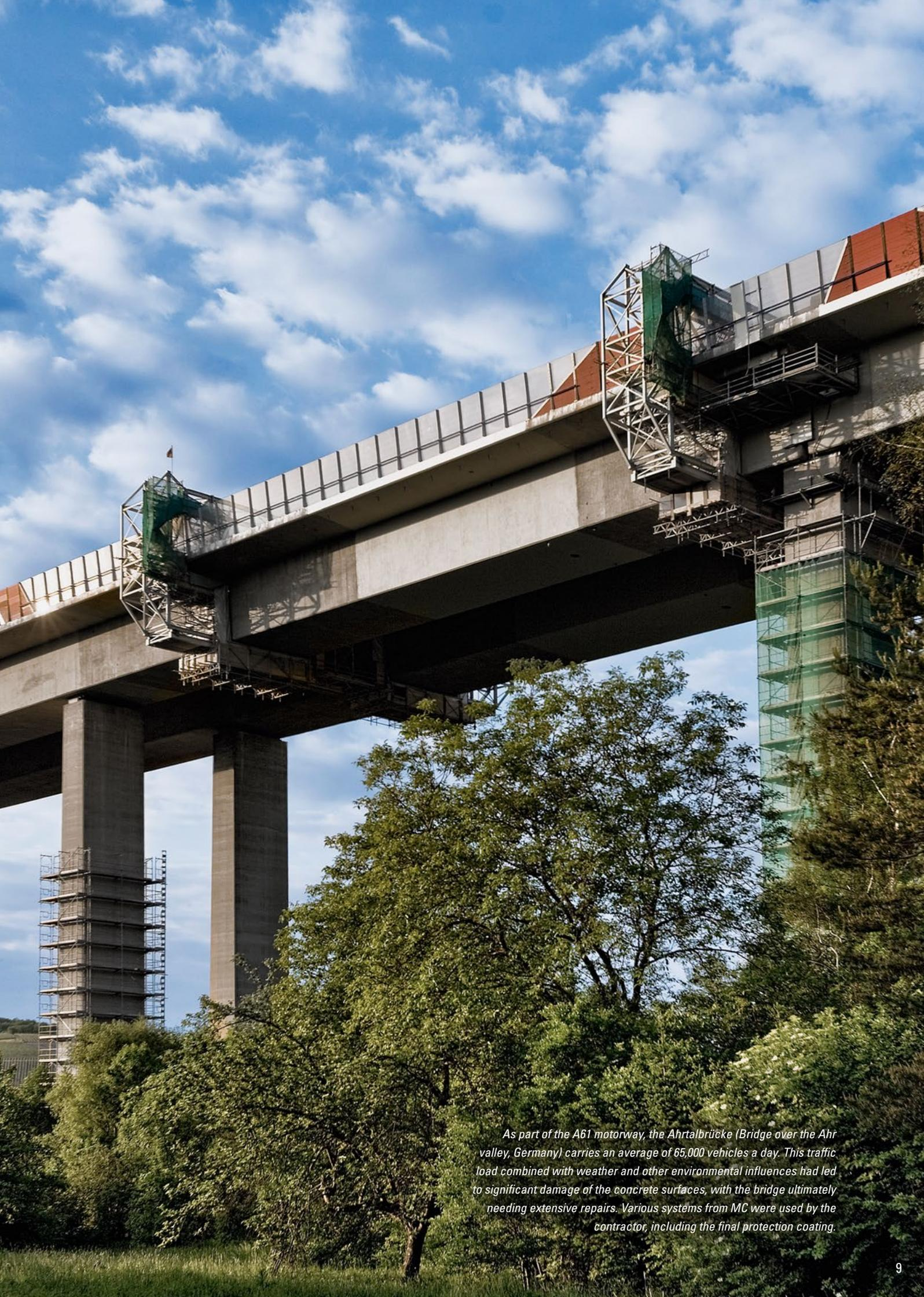
*As part of the A61 motorway, the Ahrtalbrücke (Bridge over the Ahr valley, Germany) carries an average of 65,000 vehicles a day. This traffic load combined with weather and other environmental influences had led to significant damage of the concrete surfaces, with the bridge ultimately needing extensive repairs. Various systems from MC were used by the contractor, including the final protection coating.*
