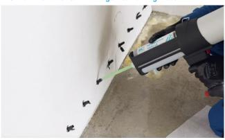
Wide area injection with MC-Fastpack 2700 via MC-Hammer Packer LP 12 into a damp component
