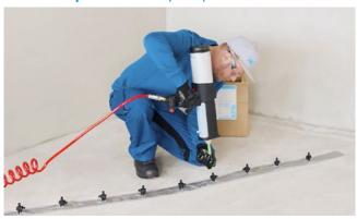
Crack injection with **MC-Fastpack 2300 top** via **MC-Hammer Packer LP 12** into a damp component
