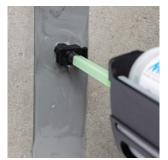
3. Insert mixer nozzle in the packer inlet spigot. Hold firmly in position and press trigger to inject.
