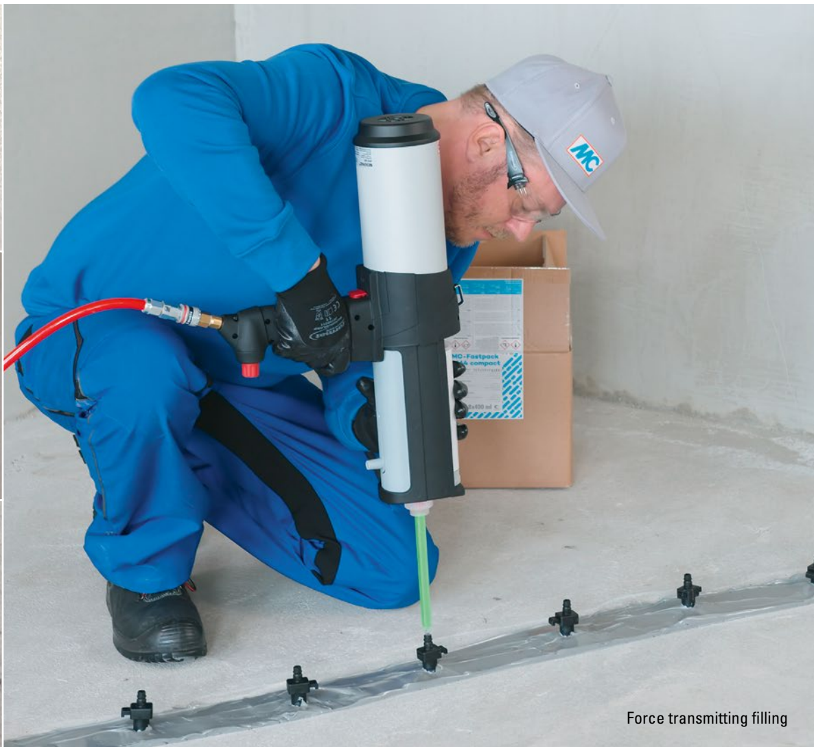
Crack and joint filling
