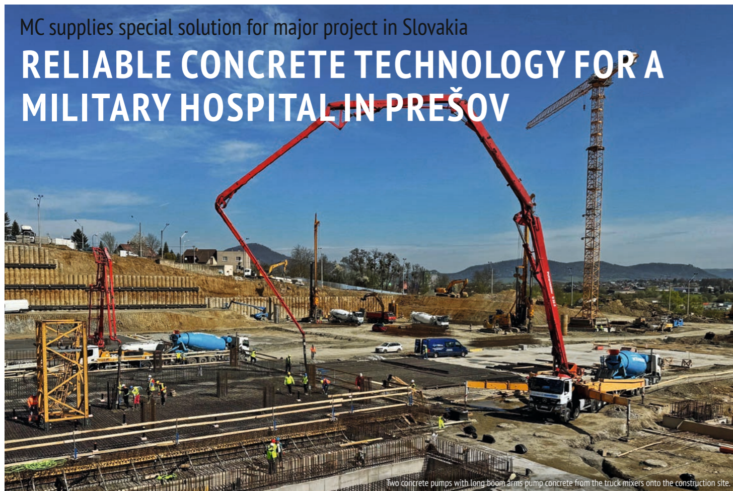
Two concrete pumps with long boom arms pump concrete from the truck mixers onto the construction site.
