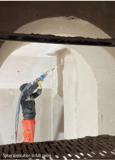
Spray application in full swing
