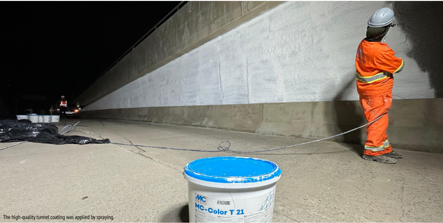
The high-quality tunnel coating was applied by spraying.
