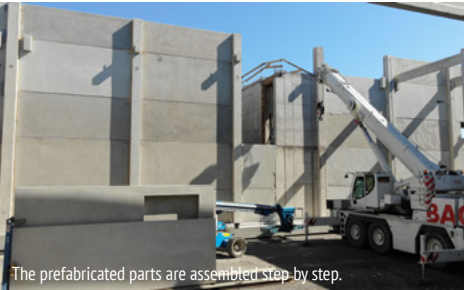
The prefabricated parts are assembled step by step.
