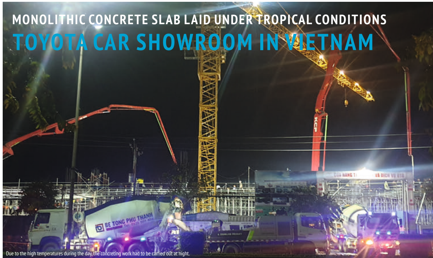
Due to the high temperatures during the day, the concreting work had to be carried out at night.
